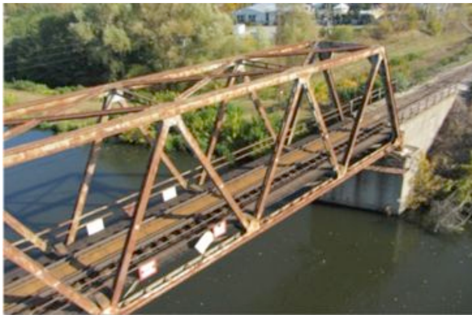
Figure 6: Railway steel bridge analysed for inspection purposes
