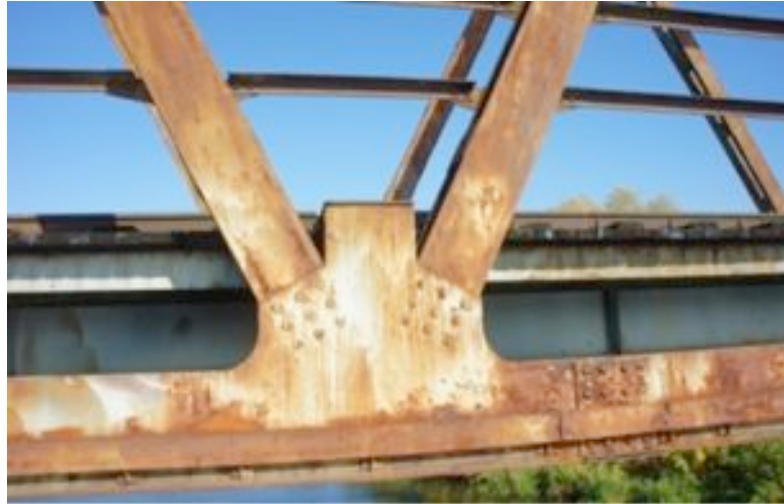
Figure 7: Detailed view of structural joint
